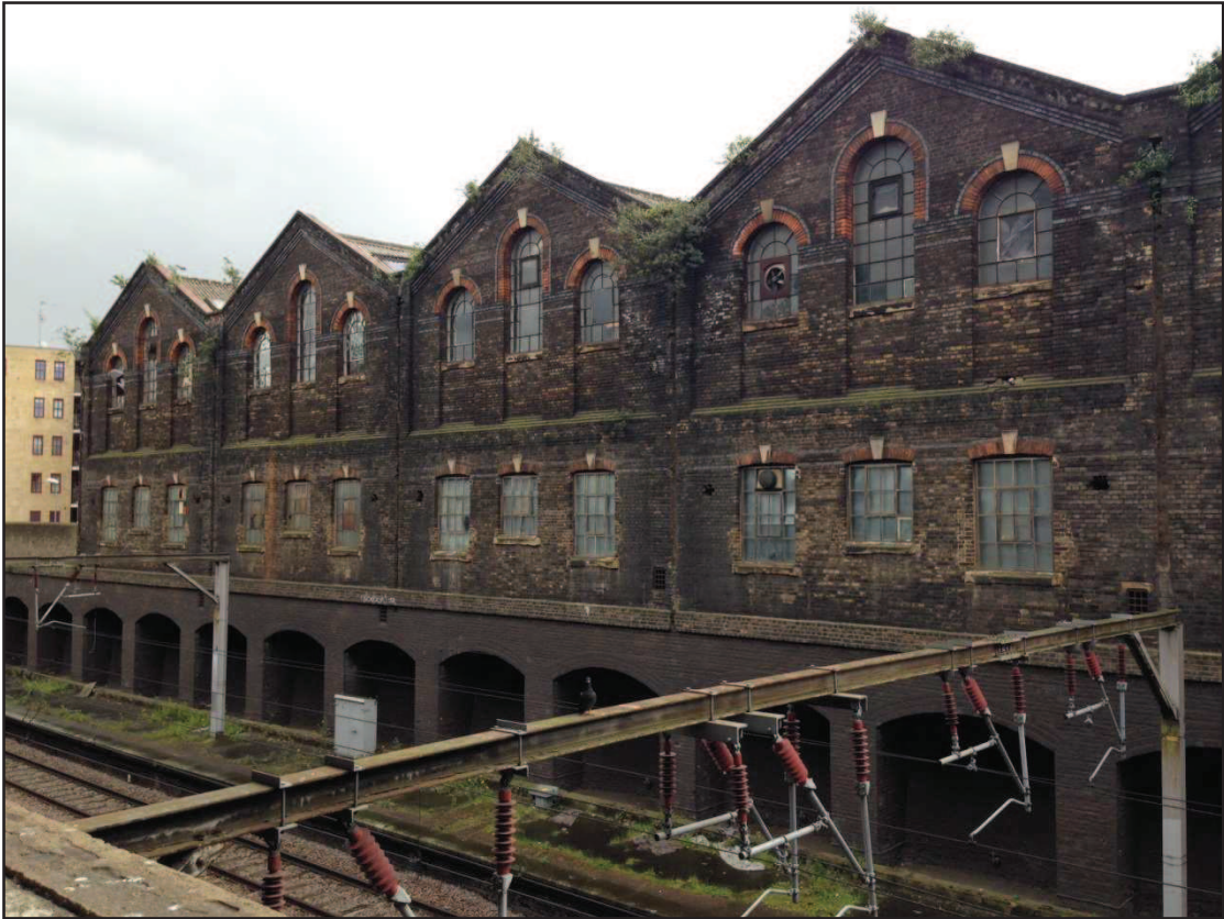
Figure 5: South-eastwards View of the Existing North Facade
